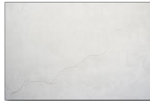
Hairline Cracks
